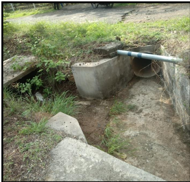
Tunnel collecting rain water for harvesting near Administrative building
