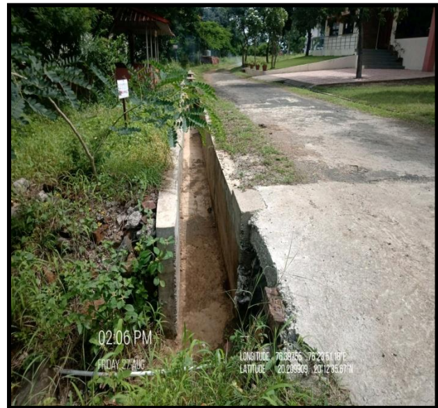
Tunnel collecting rain water for harvesting near Administrative building
